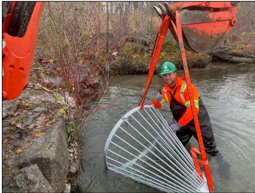
Figure 1: Installation of Beaver Cones at Dufferin Islands
