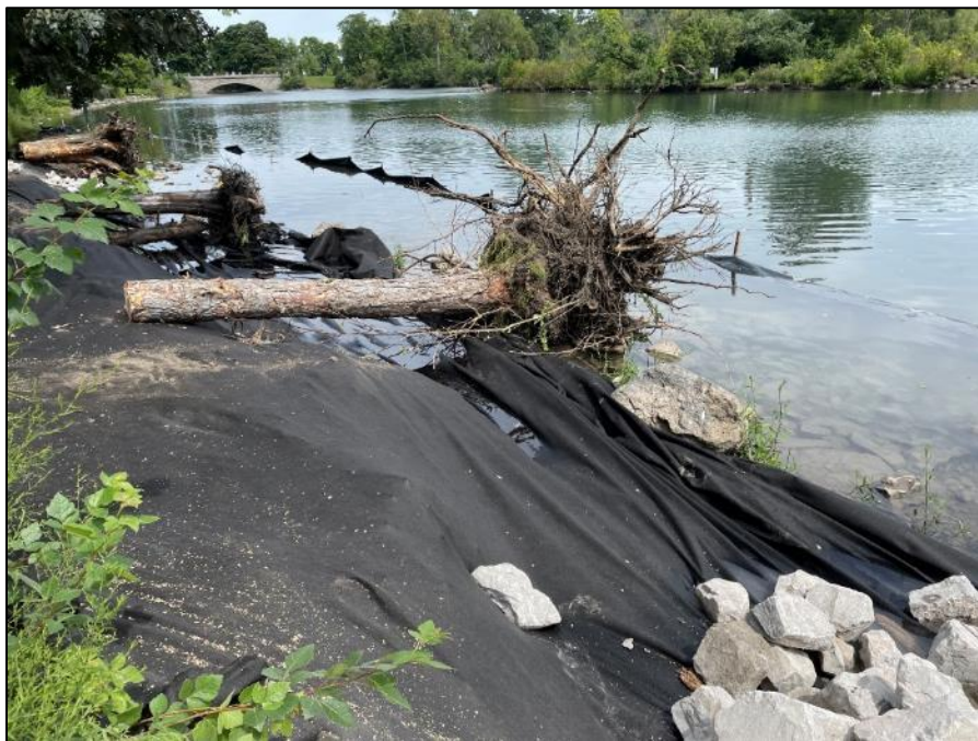
Figure 5: Installed root wads as part of bioengineering
