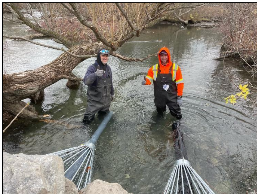
Figure 2: Installed Beaver Cones at Dufferin Islands
