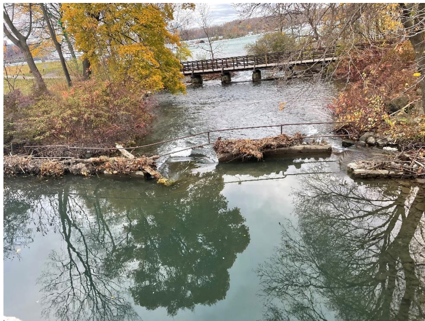
Figure 17: Failure of Weir #12 at outflow of Dufferin Islands – November 2023
