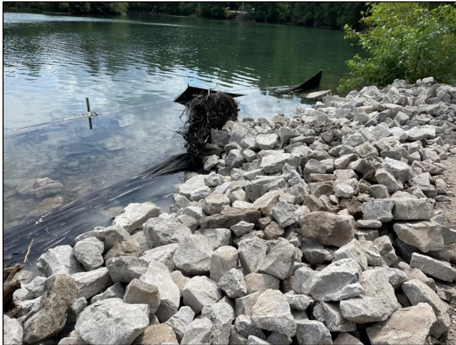
Figure 6: Rootwads anchored with rip rap
