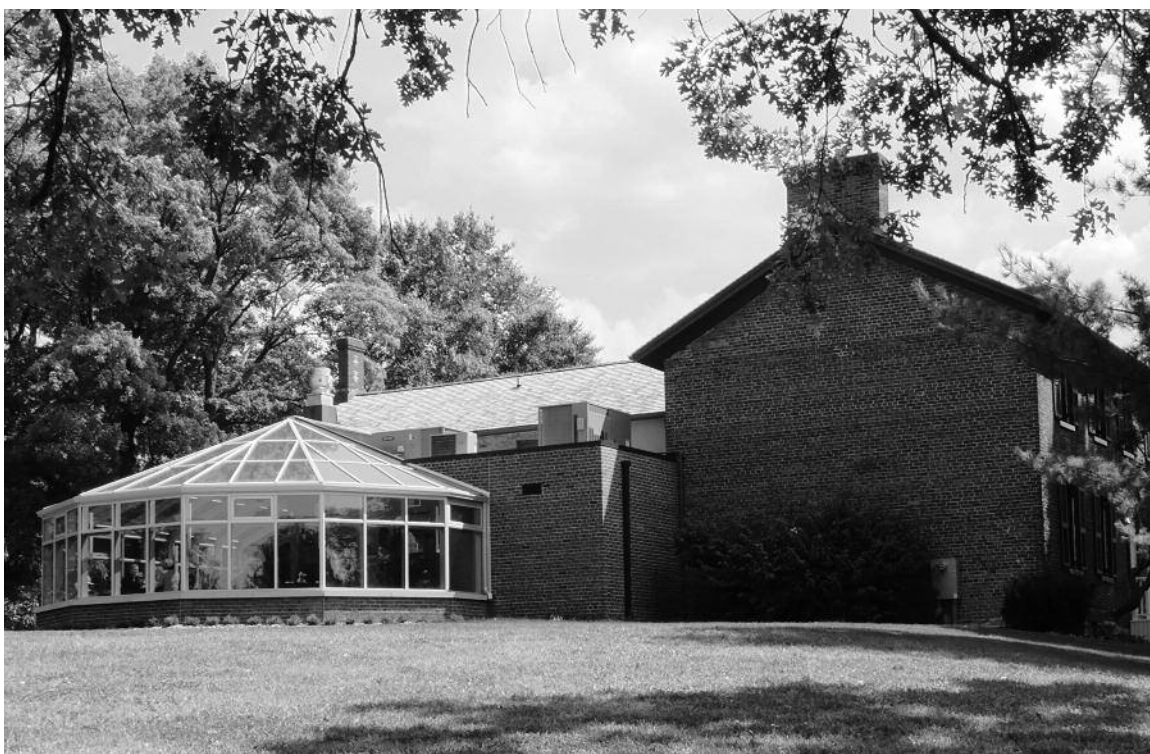
McFarland House New Tea Room Conservatory, 2011
