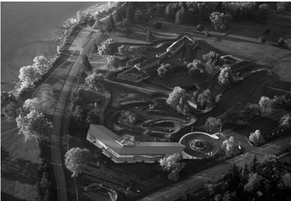
Aerial View of Old Fort Erie Vision Centre, 2011
