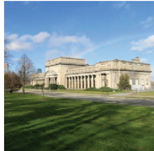
TPGS Powerhouse and Forebay
