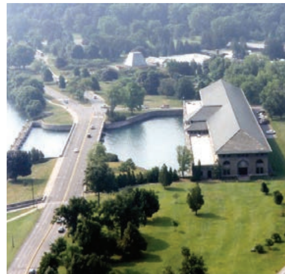
CNPGS (Rankine) Power Station and Forebay
