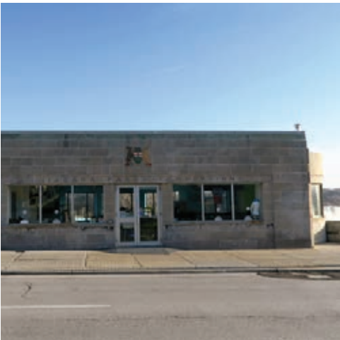
Clifton Gate House
