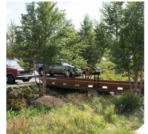
Stormwater management structure (St. Louis USA)
