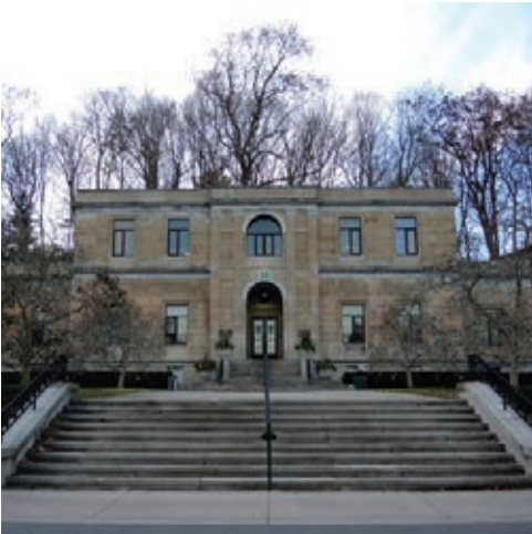
Administration Building (former)
