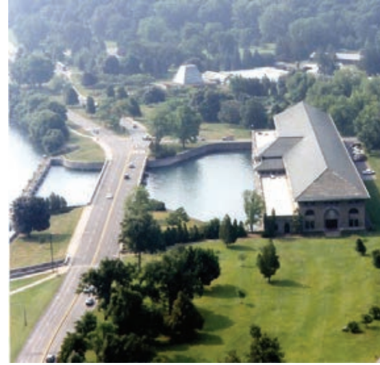
CNPGS forebay and bridges
