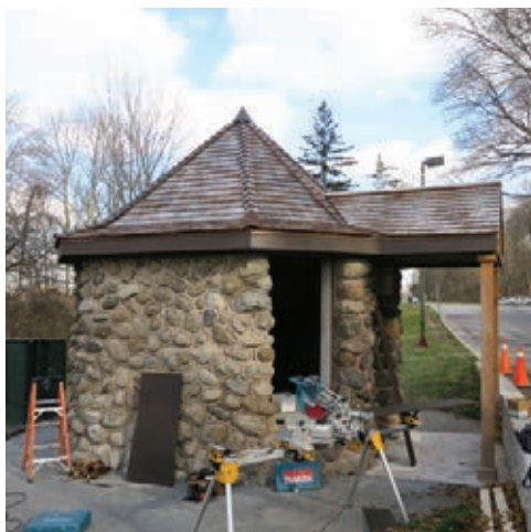
Dufferin Islands Police Hut (Cobble Shelter)
