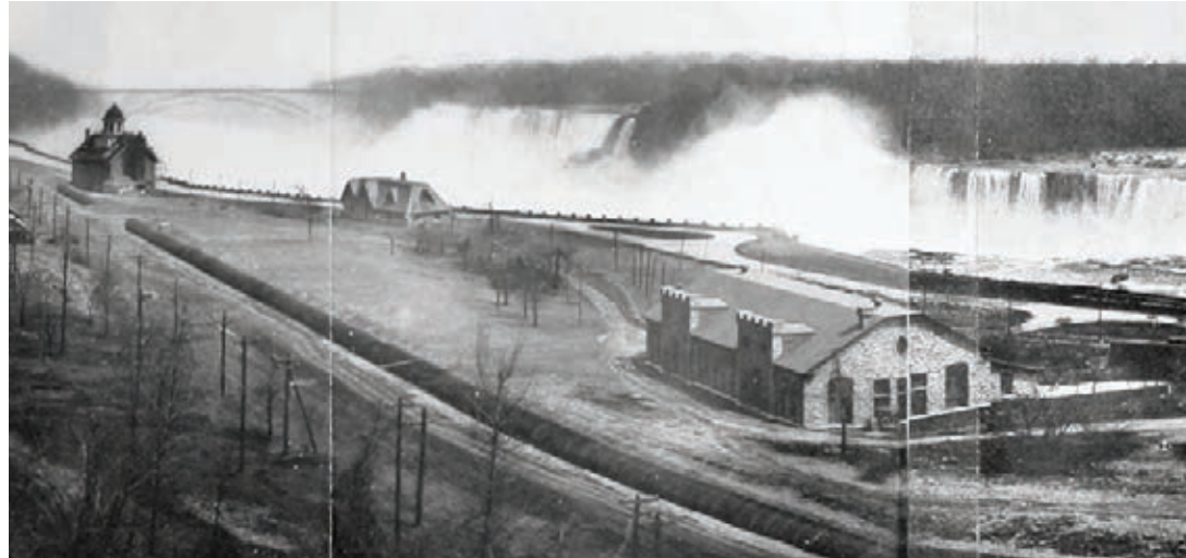
Promenade, Electric Rail, Table Rock House, and Niagara Falls Park and River Railway Company Power House (demolished), 1921
