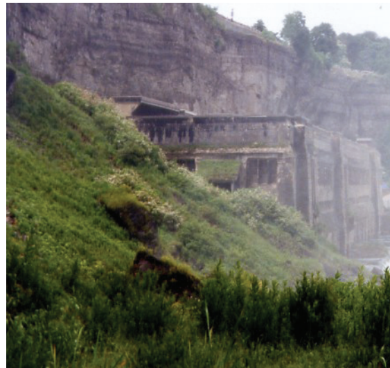
Gorge looking north towards OPGS Power Station
