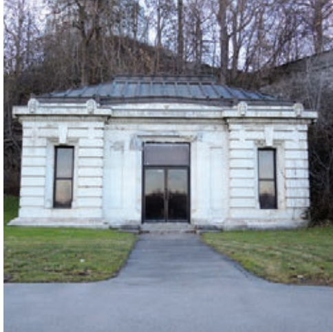
Tunnel Access Building (OPGS Elevator Building)
