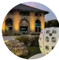
Niagara Parks Power Station + Tunnel
